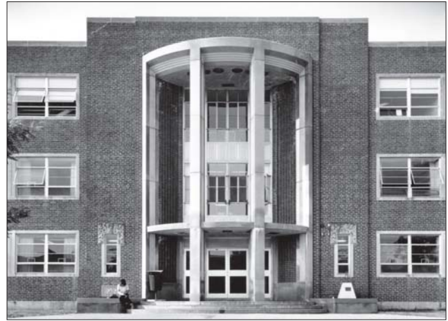
Figure 15. Kingsbury Hall, University of New Hampshire.
